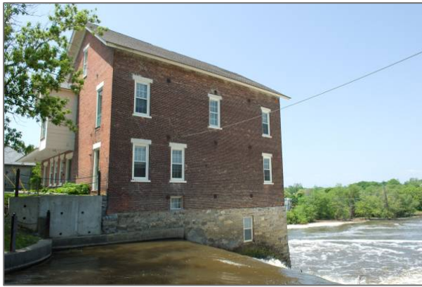
Norton Grist Mill – ‘High Rent’ Property; Location Directly on the Basin
